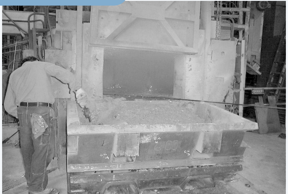
Operator tending a typical aluminum melting furnace.
